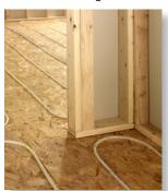
floor, heat radiates evenly up through the floor. providing quiet, even warmth while using less energy. SSS 🤌 🤌
