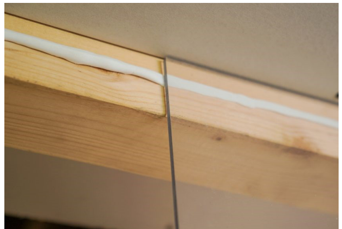
Plexiglass used to illustrate how gasket seals the gap where the wall drywall would be installed
